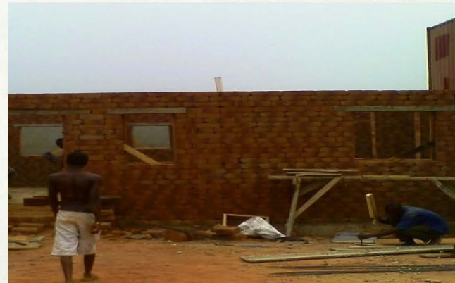
A school being built with Natural Crete bricks and blocks.
